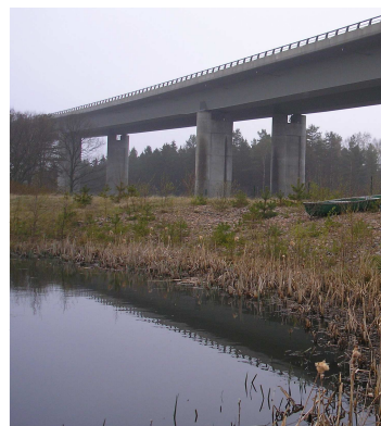
Fig. 4. Road runoff detention pond in the western part of Sweden.
