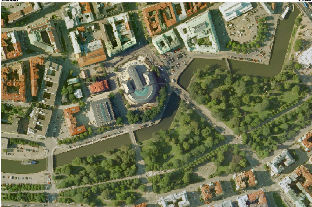
Illustration 18. The central part of Vallgravsstråket - Rosenlundsbron to Kungsportsbron
