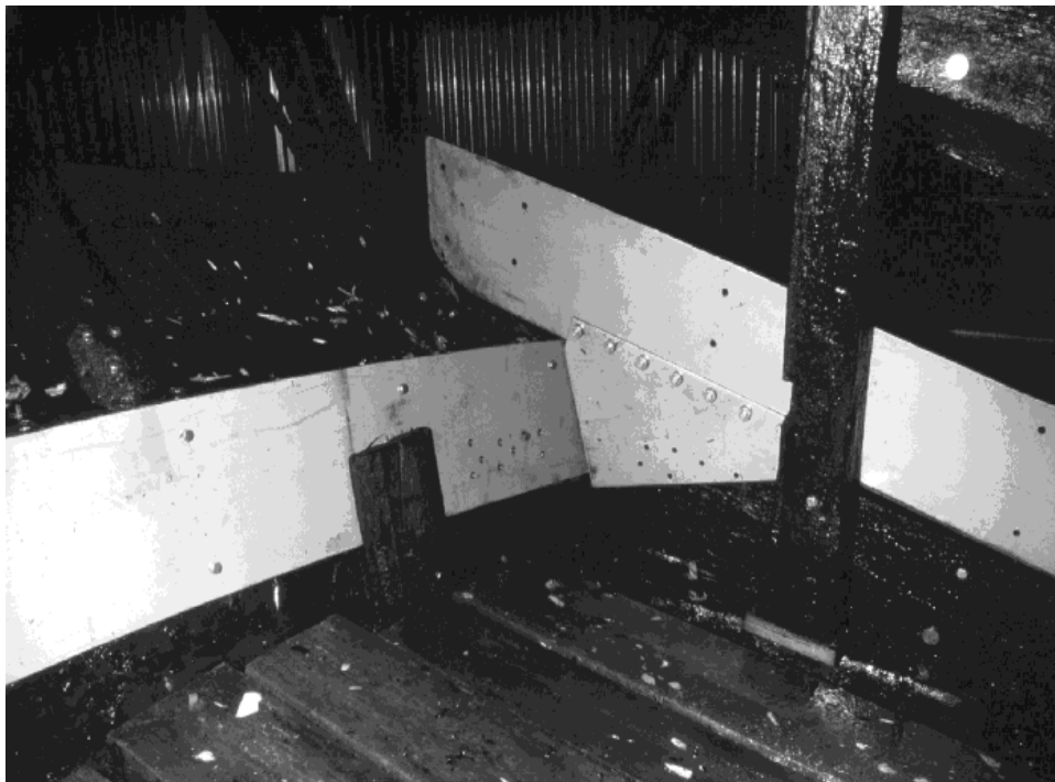
Figure 3-18 The steel construction, detail (photo: Björn Hedin)
