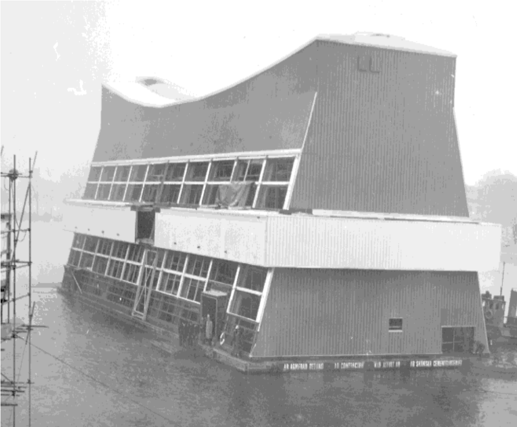
Figure 3-7 The Vasa pontoon with the superstructure approaching the museum site (photo from the archive of the Swedish National Maritime Museum)
