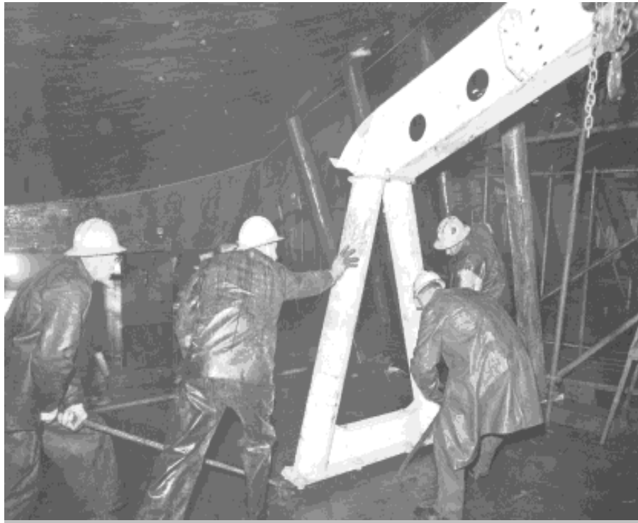
Figure 3-11 Mounting of the cradle in the pontoon superstructure (photo: Göran Sallstedt)
