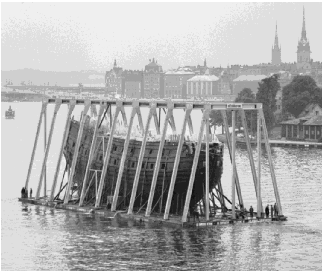
Figure 3-6 The pontoon with the concrete beams leaving the dry dock (photo from the archive of the Swedish National Maritime Museum)
