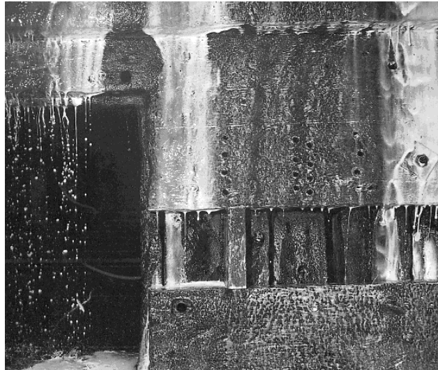
Figure 4-21 Foam on the surface of the hull produced by the spraying of the preservation liquid (photo: Göran Sallstedt)
