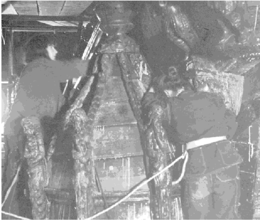
Figure 4-26 Removing loose dust with a vacuum cleaner (photo: Sven Bengtsson)
