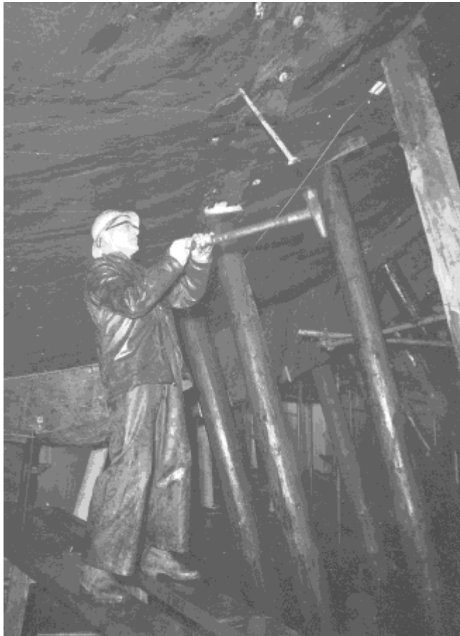
Figure 3-15 Inserting bolts into the original bolt holes (photo: Göran Sallstedt)
