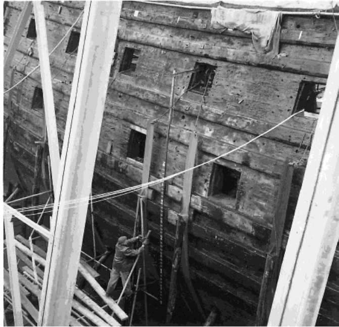
Figure 3-4 Props supporting the Vasa hull on the pontoon (photo: Gerhard Bauer)
