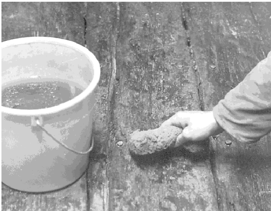
Figure 4-27 Cleaning the dirty surface with a moistened genuine sponge (photo: Sven Bengtsson)
