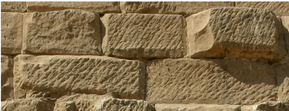
Fig. 110: Detail of the undressed section of the northern gate at Karnak. The rough faces of the stone blocks show diagonal, elongated chisel marks that are identical to the pattern surrounding the crown of Arsinoë in cat. no. 26L. The relief of the decorated faces (N-S) dates to the reign of Ptolemy III. Photo by the author.
