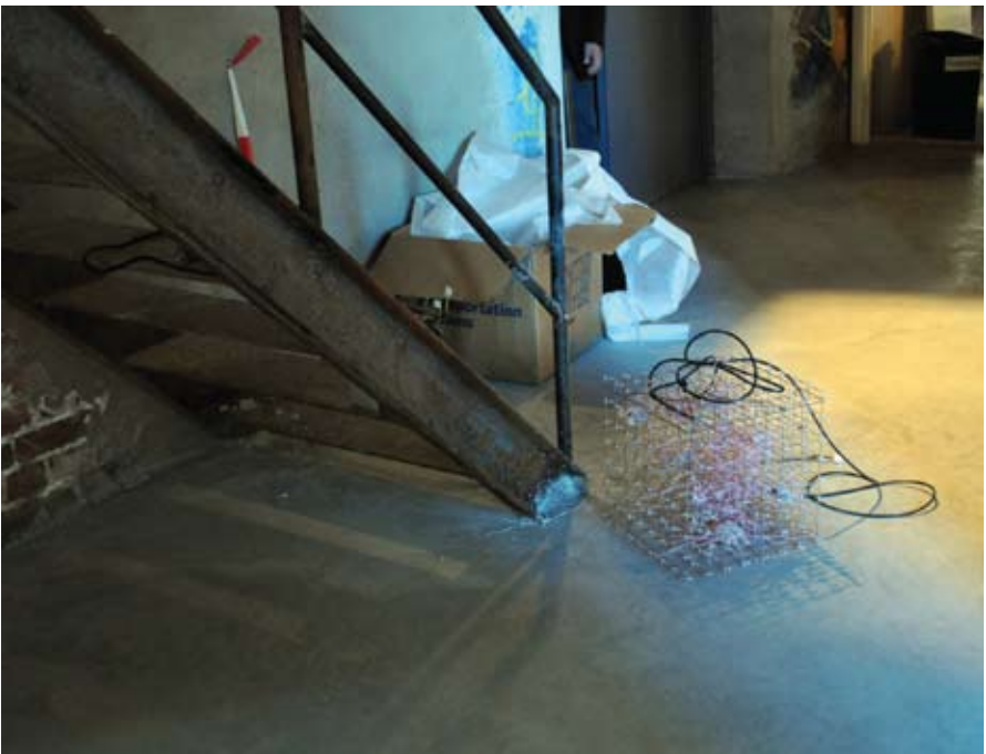
Images 71-72 : Construction at Röda Sten, 2010
