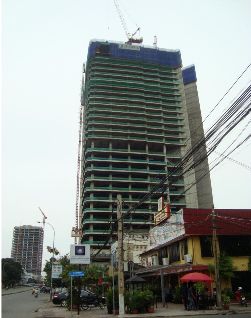
Construction of high-rise buildings in central Phnom Penh
