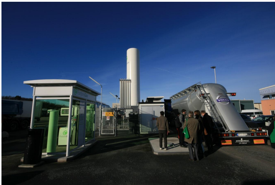
Figure 12, Filling station for liquefied methane/ Stigs Center Gothenburg. (Picture: Sporer)
