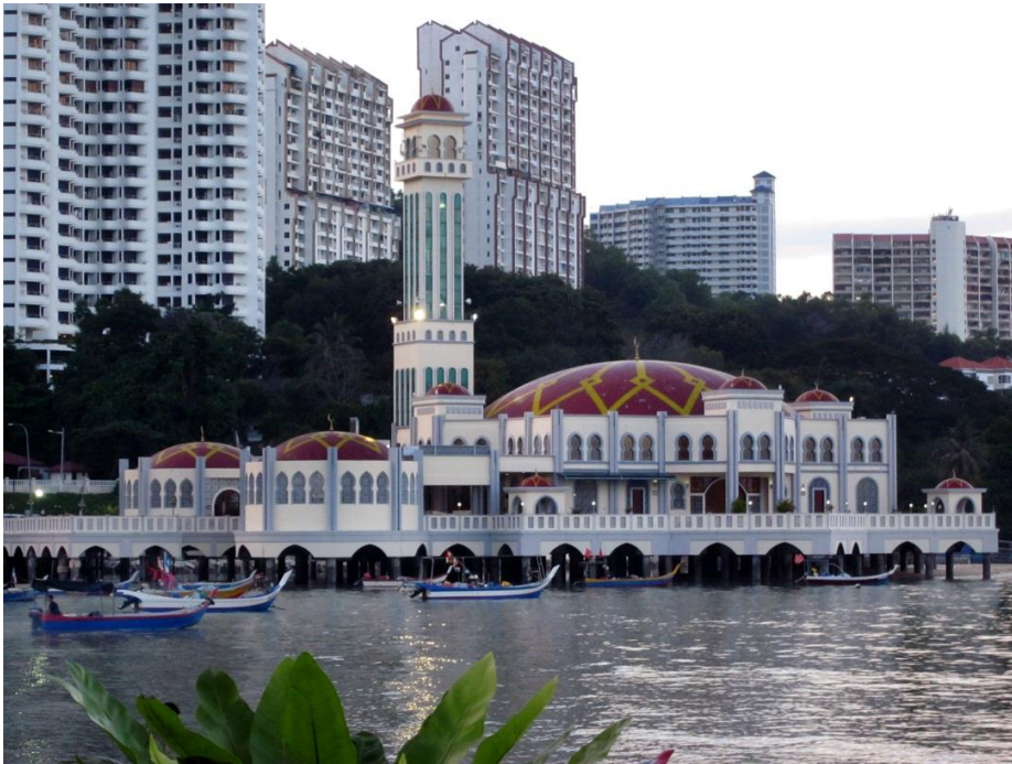
Figure 13. The Tanjung Bungah floating Mosque, 2010.
