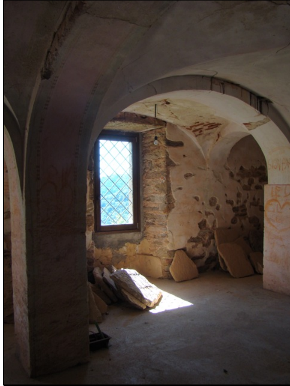
Figure 8: la Trappa, restorations underway
