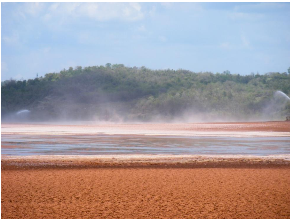
Picture 4.3: close up of the red mud lake, with sprinklers trying to keep it moist. But due to wind dust plumes are forming.
