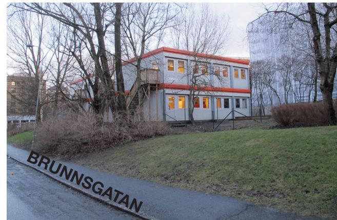
The site viewed from Brunnsgatan, The building behind is Annedalsskolan which is being renovated and therefore covered with fabric.
