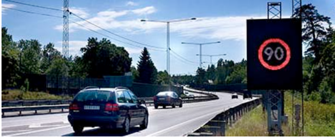
Figure 5: Digital road signs at E18 in Sweden (DN.se, 2008)
