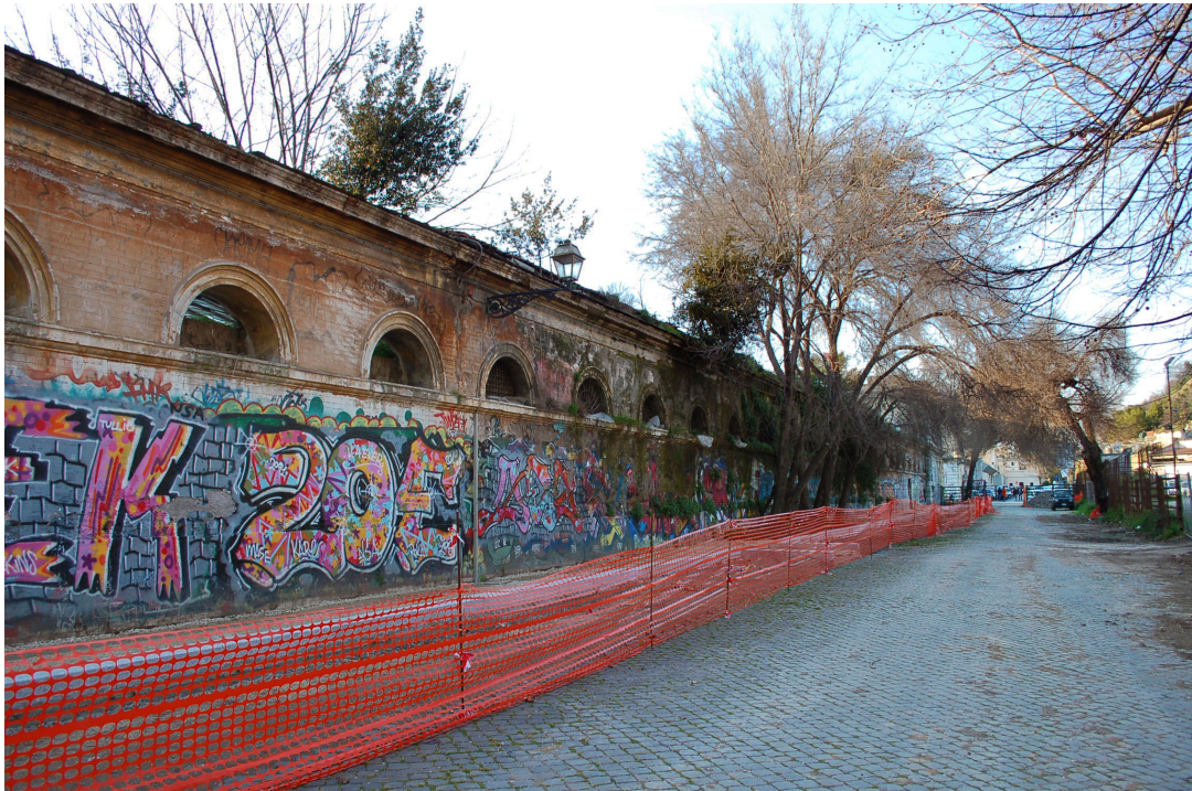
Fig. 11 Exterior of the slaughterhouse awaiting restoration
