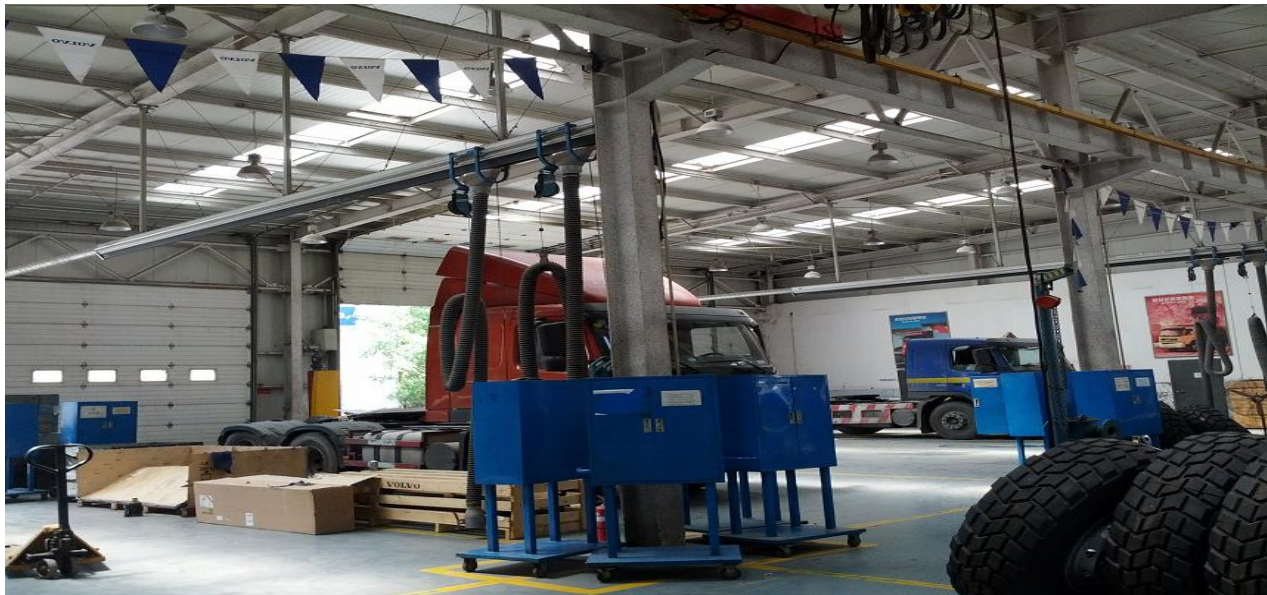
Figure 7 Volvo Dealer workshop located in Borås city in Västra Götaland
