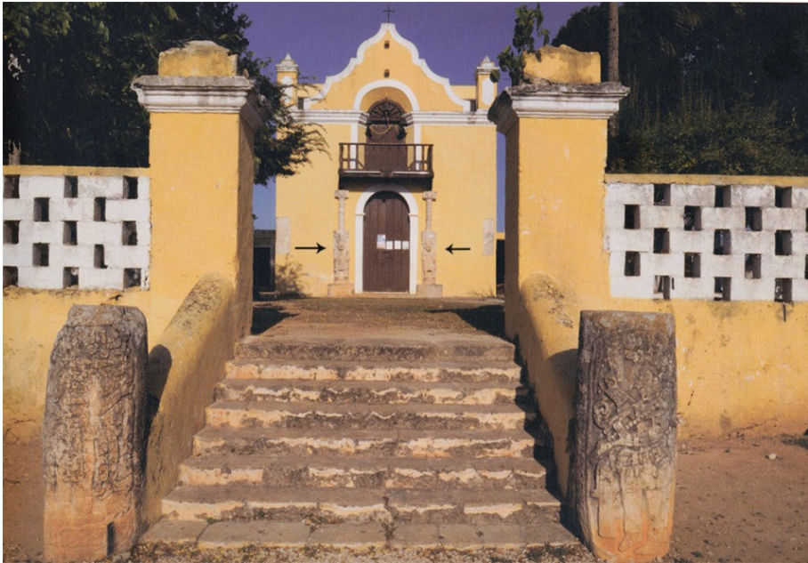
Figure 31. Entrance step to the Santa Bárbara chapel in Yucatán. The Maya Stelae are on the first level. Two sculptures are on the second level on either side of the chapel door.
