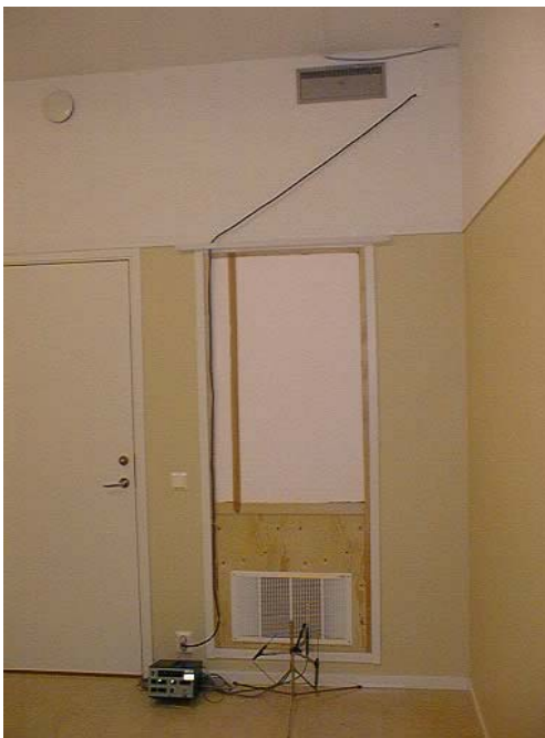
Figure 72. In the left picture the white diffuser at 0.2 m height and the grey squared mixing grill to the right side at 2.9 m and the white round exhaust at 2.9 m to the left. The right picture shows the air supply to the room from the corridor side.
