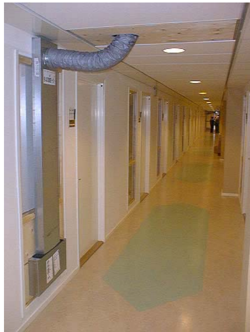
Figure 72. In the left picture the white diffuser at 0.2 m height and the grey squared mixing grill to the right side at 2.9 m and the white round exhaust at 2.9 m to the left. The right picture shows the air supply to the room from the corridor side.
