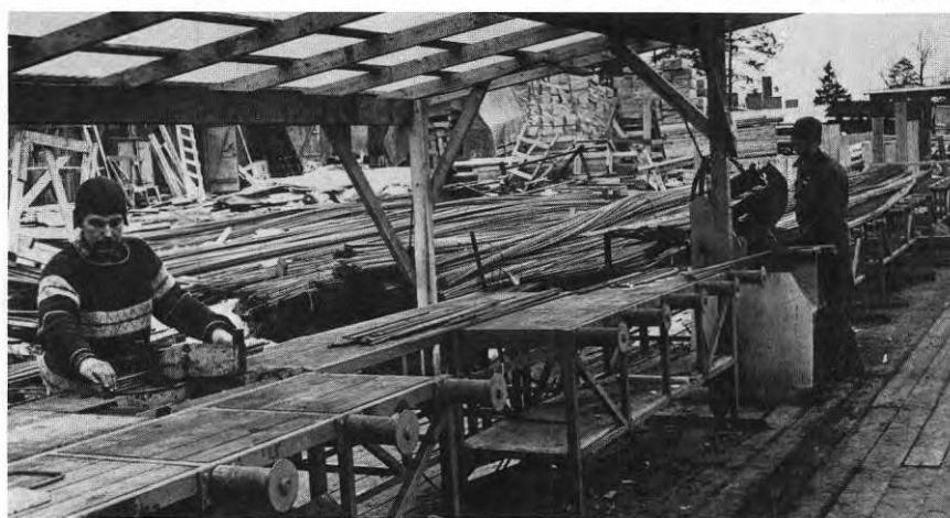
FIG. 1. At the modified reinforcement station, the work of shearing and bending the rods is done at the same height. The two operations can also be done at the same time. The work bench slopes in the direction of the steel transport, and the rollers have ball bearings.
