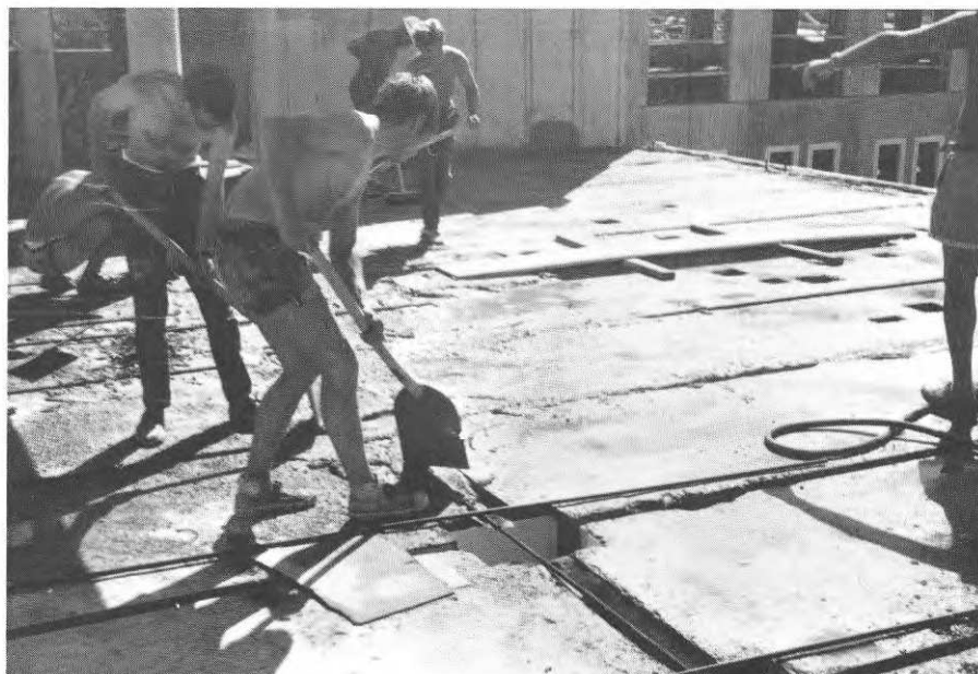
FIG. 42. Bruket skyfflas ned i fogarna. Slurry being shovelled into the joints.
