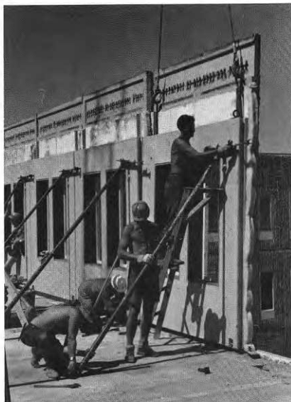
Fixing of ties to external wall panels.
