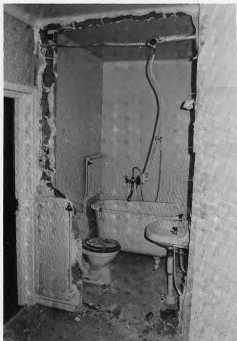
Figur 4.19 Badrum under rivning Jakthunden 4
