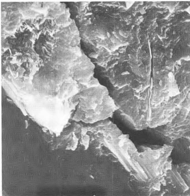
Oskadad betong, skarv cement/sandkorn
