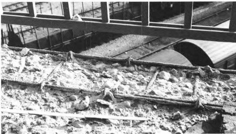
Fig 2 Saltskador i modern betongbro, Stockholm (B Steorn)
