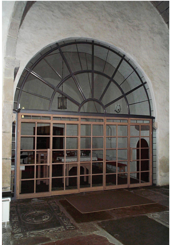
Figure 1. A reversible glass wall between the nave and the tower in Grötlingbo church, Gotland. Photo by Tor Broström.
