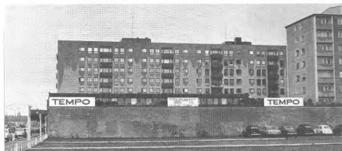
Fig. 14. The windward side of a building immediately after a light shower. Note the uneven distribution of the rain.
