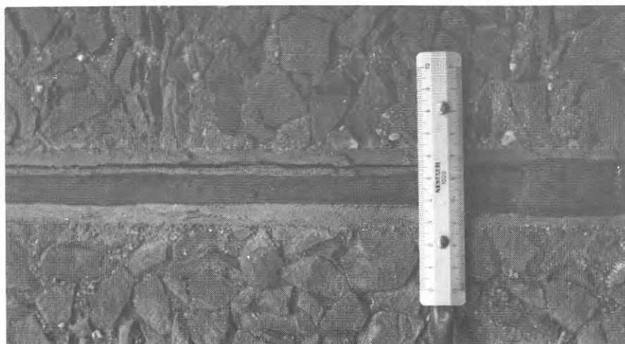
Fig. 44. Joint made up of resilient jointing compound based on polysulphide laid between two buildings constructed with different kinds of brick. The joint has sagged against the brick of lower density.
