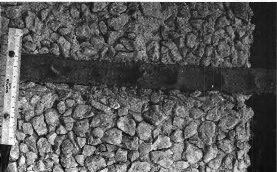
Fig. 82. Vertical joint between room-size concrete sections containing pointed-over skin-forming oil-based jointing compound, photographed after 12 years in a partially shaded courtyard wall. The paint and the jointing compound have formed a skin with a thickness of up to 0.5 mm. There are isolated cracks in this skin.
