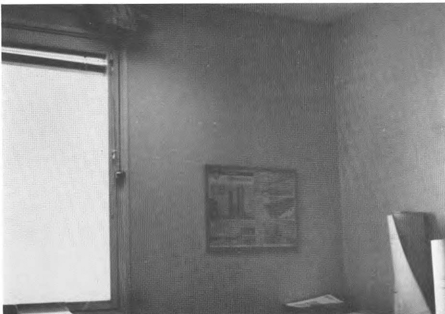
Fig. 51. Window showing early damage to paintwork on the wood near the joints. The joints between the casement and the frame, the joint around the plug and the joint between the flashing and the frame has cracked, allowing water from rain and melting snow to penetrate. Note suction into the end grain into the bottom casement timber. The sharp edge on the bottom frame piece is not completely covered by paint.
