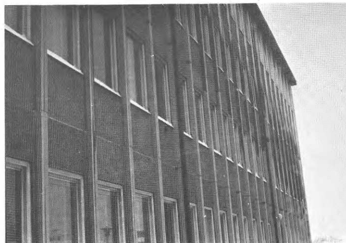
Fig. 16. A concrete facade immediately after a snow shower. The photograph gives an example of the distribution of precipitation on the lee of a building. Note the effect of the vertical pattern. Snow has collected at the bottom of the windows.
