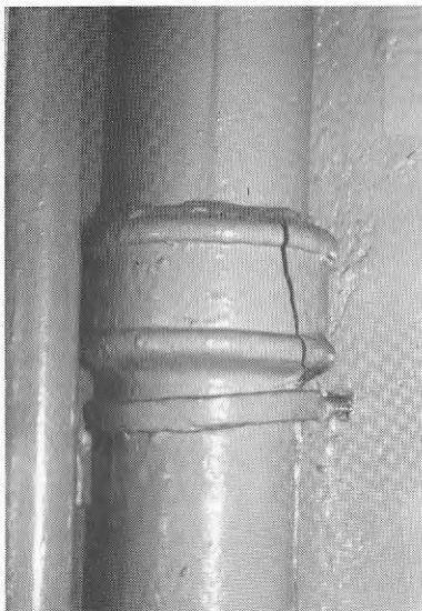
Figur 6.3 Sprucken avloppsstam
