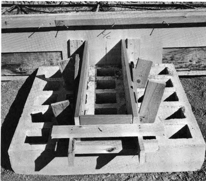
FIG. 1. Photo showing a grid with formwork for the pedestal.
