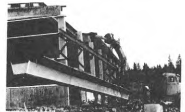
Photograph 2. Cassette being erected.
