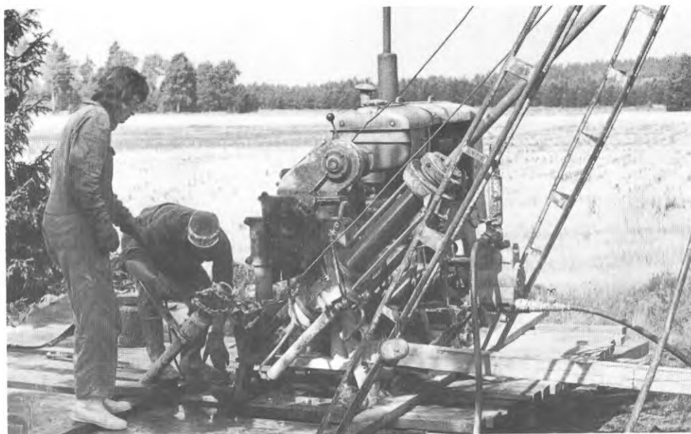
FIG. 7. Kärnborrning i Haninge (Craelius D 750). Core drilling in Haninge (Craelius D 750).
