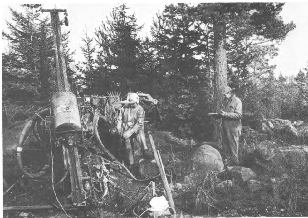
FIG. 11. Slående sonderingsbörning med ROC 601 i Forsmark. Borrsjunkningen registrerades såväl automatiskt som manuellt. Percussive investigation drilling with ROC 601 at Forsmark. The penetration rate is recorded both automatically and manually.
