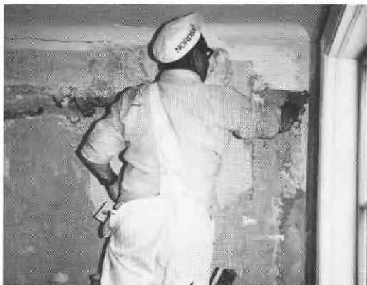
FIG. 15.4. Bredspackling.
