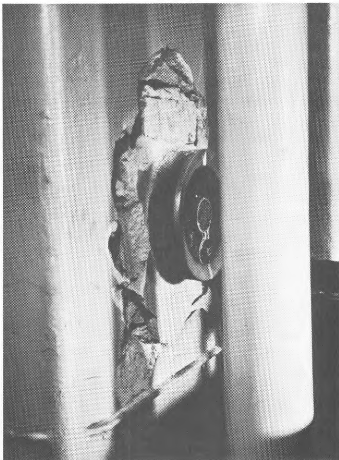
FIG. 13. Inmurad dragregulator i murstock.
