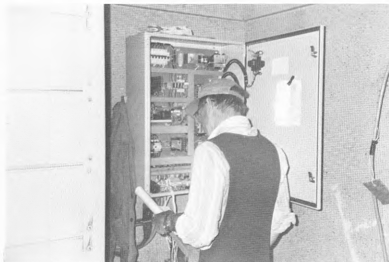
Fig 229. Installation hissmaskineri
