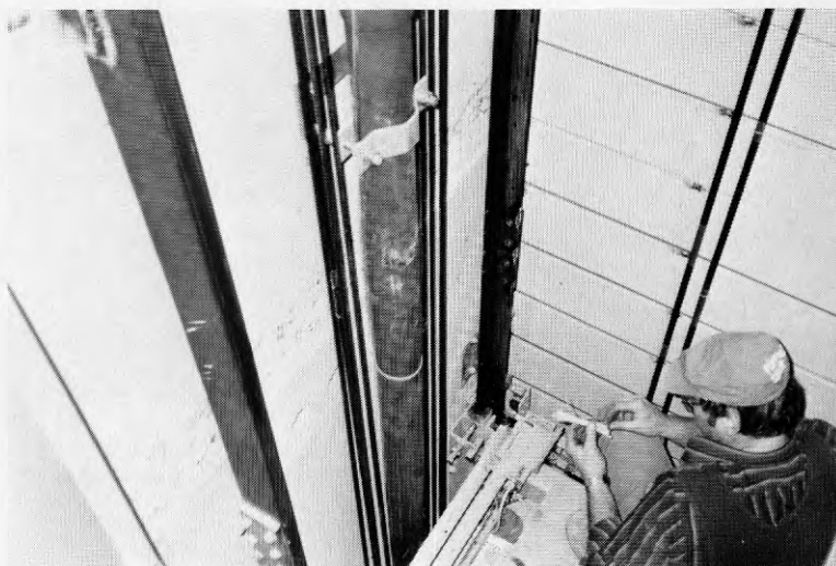
Fig 228. Installation i schakt
