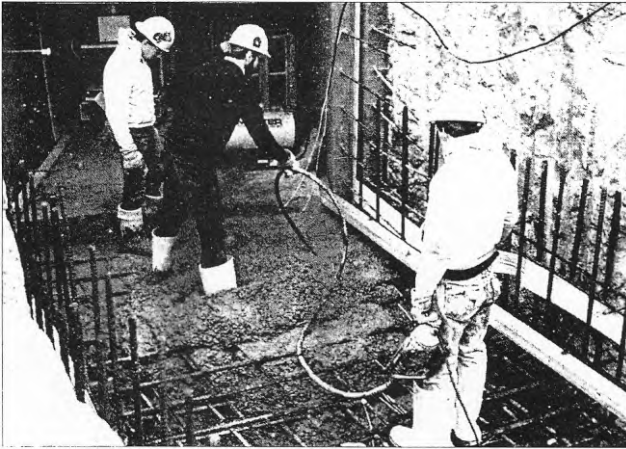
Figur 7.10.1:7 – Installation of optical fibers in the formwork
