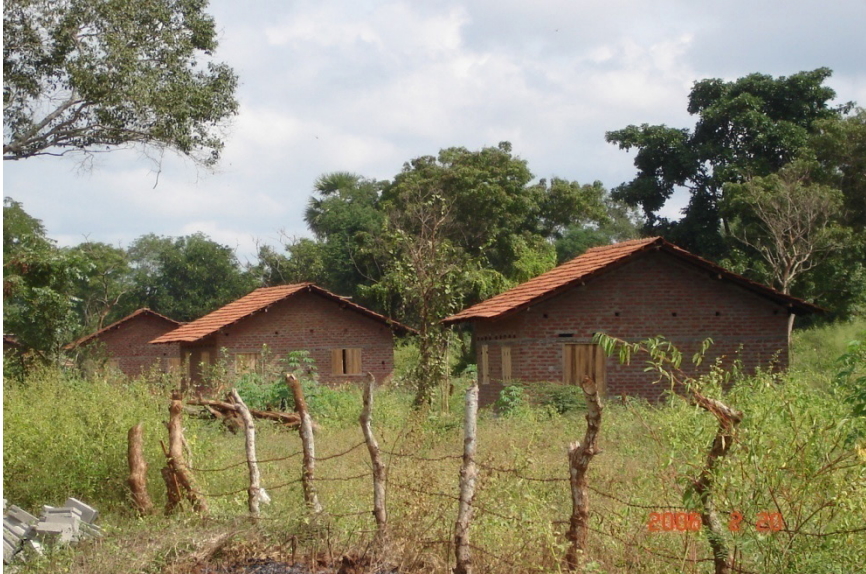
Figure 9.4. Newly Built Houses in Paleo Oruwa -Vavuniya South with assistance given by the Government Resettlement Scheme- 2005
