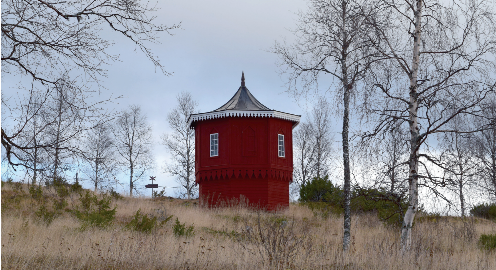
Figure 19. A reconstructed pivot, originally built in 1859 to rotate wires from a waterwheel controlling the waterlevels in the mine.
