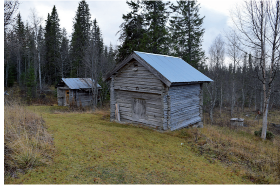
Figure 23. Authenticity in terms of original roofing has been negotiated in order to avoid future costs.
