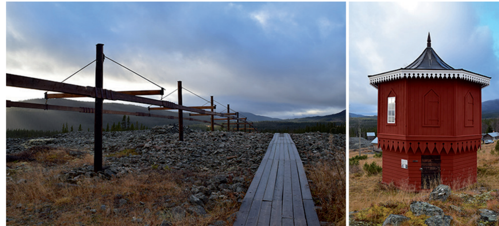
Figure 4. Reconstructed flat rod system and pivot originally built in 1859.
