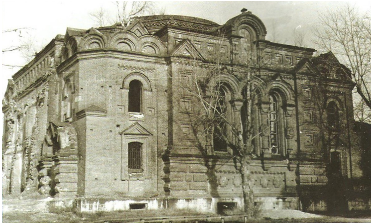
Fig. 3. The church of the Ascension, 1980s (approximately). The church was built in 1913 as a new monastery church (there is one more, an older and smaller church, on the right side, not visible in the picture). Somewhere in the Soviet times, the church was deprived of all the domes and even the narthex, on the left. Now the church is restored outside.
