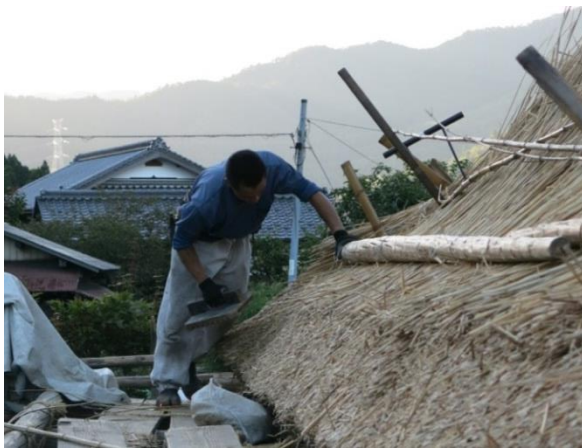
Fig 10. Smoothing the surface.
