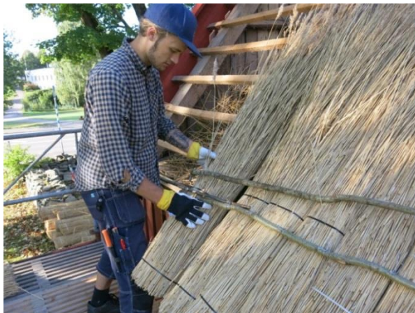
Fig 18. Placing the bundles on the truss.
