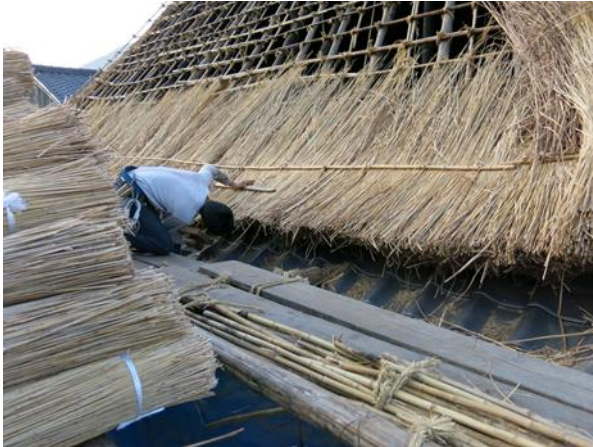
Fig 8. Making the first layer.
