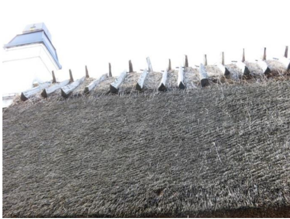
Fig 22. The cut roof surface.
