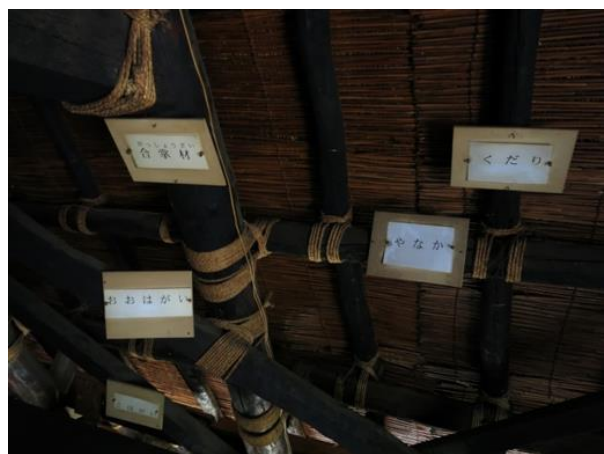
Fig 68. Name tags on the roof structure.
