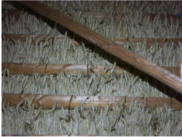
Fig 37. The smithy roof from inside.
