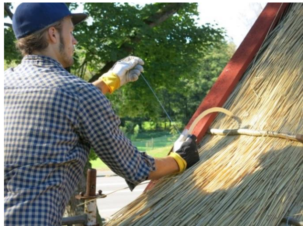
Fig 19. Fixing with galvanized steel thread.
