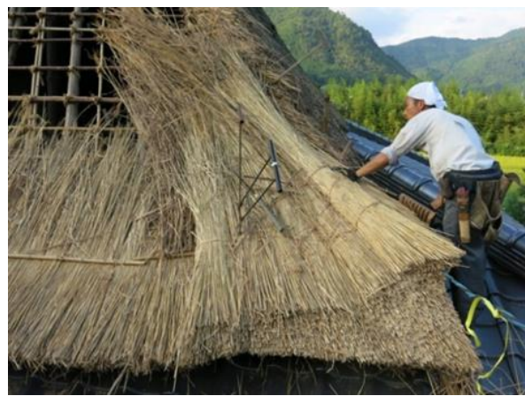
Fig 11. Making the corner and the next layer.
