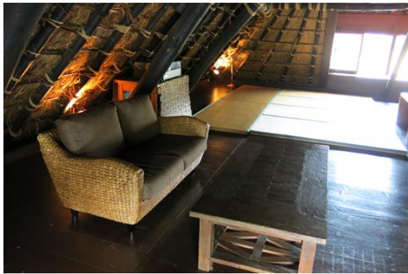
Fig 33. The inn's inner roof.
