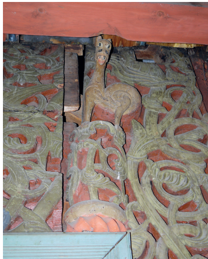
Fig. 4.8. Above , the most likely original miniature lattice truss in Nore stave church, which is located over the west portal however, hidden by the subsequent ceiling in the present porch. Below left , portal carvings without subsequent paint, that are also located over the ceiling, and not visible from the porch. Below right , the top of the portal carvings that are visible in the porch. Photo 2016.
