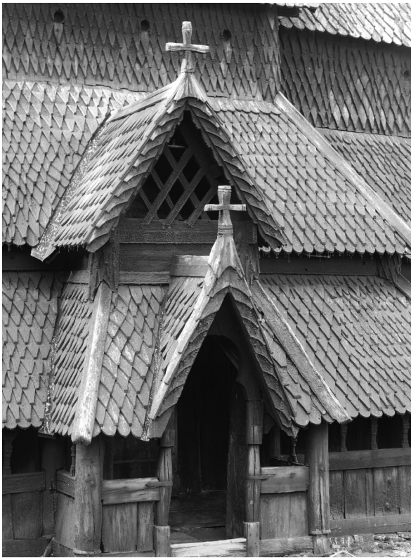
Fig. 4.7. Left , the entrance to the gallery in Borgund, and right , the bell tower in Borgund. Both have 'lattice' grids. The bell tower in Borgund is the only freestanding tower with stave construction in Norway (Anker 2005:151). The bell tower in Lomen stave church, also have lattice, see picture in Hauglid (1990:59). Photo 2016.
