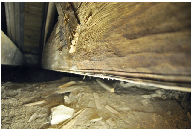
Fig. 3.13. Above , 3D scan of the scarred strut, placed towards the south wall and the window. This is the only truss were the carpenters chose to use timber which had been scarred like this, likely by lightning. They chose to expose the scar by placing it at the [west] front side. Further, it was placed in the very middle of the room, and it was well lit by the window. I interpret that this placement was intentional. Spetz 2014. Below left , the carved thin beaded curve. Photo Eriksson 2012. Below right , the black line under the tiebeam [truss 9], which marks the middle of the room. Photo Eriksson 2012.
