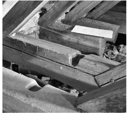
Fig. 3.11. Left 3D laser scan of the west truss [1]. Spetz 2014. Right trace from something hanging in the tiebeams [2, 3 and 4]. Photo Eriksson 2012.
