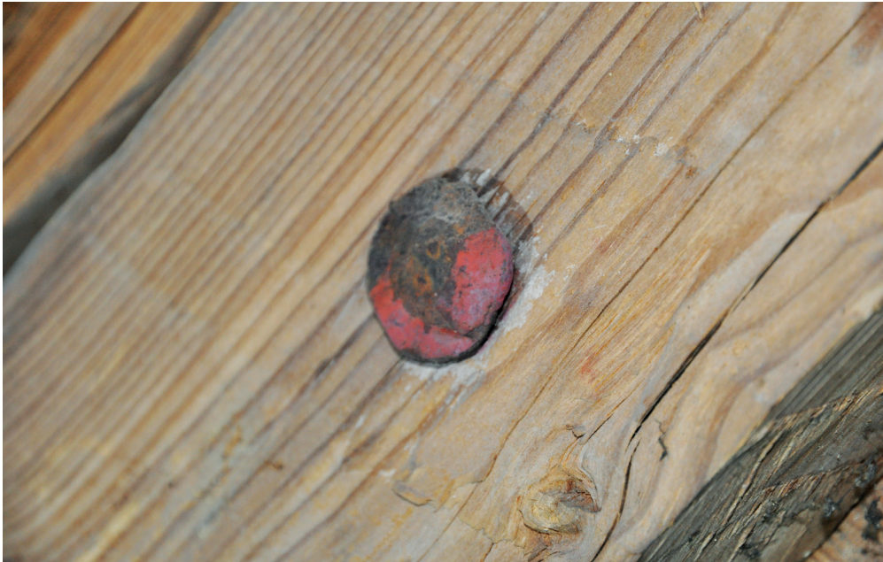
Fig. 3.9. In Mosjö church in Närke, red paint remains on an iron nail. Remains of white paint occur in many places in this roof, and in some cases traces of black (Eriksson & Borg 2014:76f, 81). The roof over the nave in Mosjö church has been dated with dendrochronology to 1214 (ibid). Photo Eriksson 2014.
