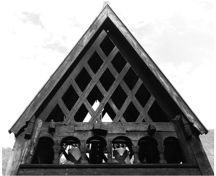
Fig. 4.7. Left , the entrance to the gallery in Borgund, and right , the bell tower in Borgund. Both have 'lattice' grids. The bell tower in Borgund is the only freestanding tower with stave construction in Norway (Anker 2005:151). The bell tower in Lomen stave church, also have lattice, see picture in Hauglid (1990:59). Photo 2016.
