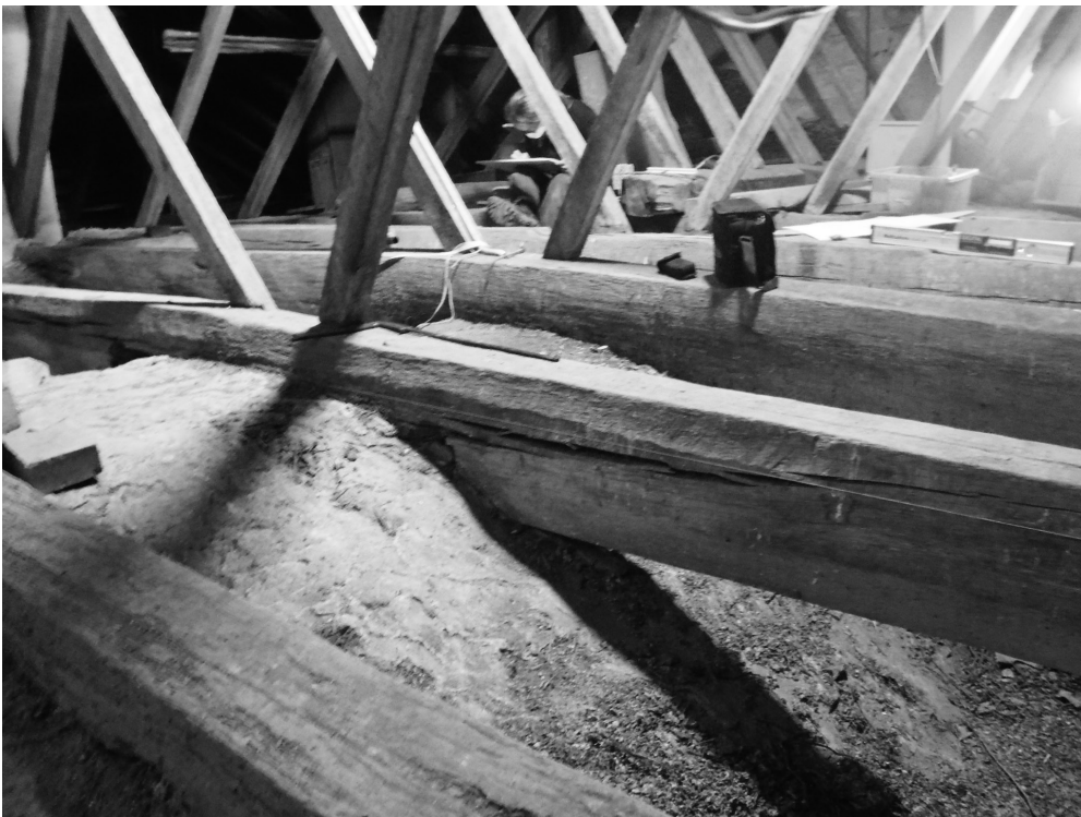
Fig. 4.19. Tiebeams and vaults in Forshem. Photo Eriksson 2011.
