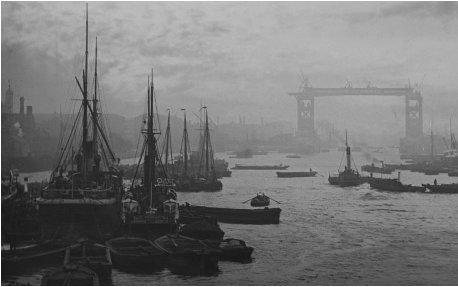
Lower Pool, with Tower Bridge under construction. This is an early photograph (1886-1894) of Thame's Lower Pool that depicts the Tower Bridge under construction and the vibrant industrial and trade activities in the city of London. Reproduction by permission of © Museum of London.
