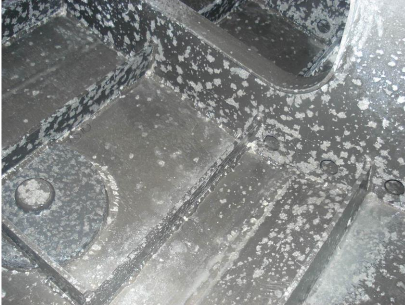
Figure 22. Common pitting corrosion on aluminium that has been caused by chlorides.
