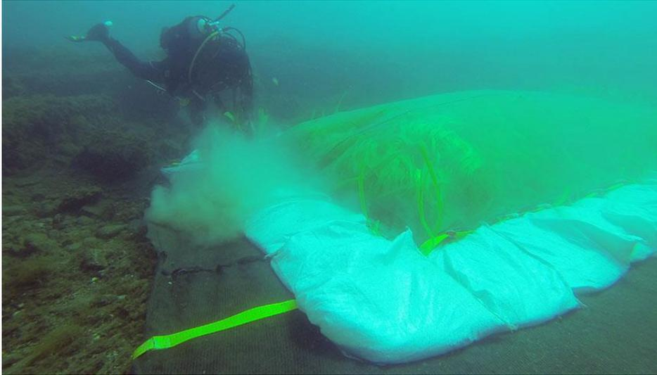
*Figure 8: Sediment trapping using geotextiles and artificial seagrass. (SASMAP Consortium, n.d.)*
