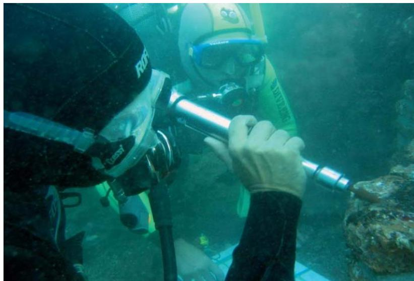
*Figure 10: Removing biological encrustations using a pneumatic microgrinder in Baiae. (Petriaggi and Davidde, 2012)*
