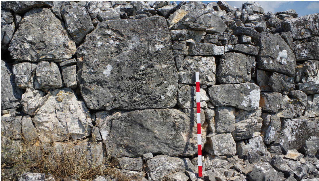
Figure 4.13: Rohpolygonal masonry, first phase enceinte at Vlochós, Thessaly. Photograph by Robin Rönnlund.
