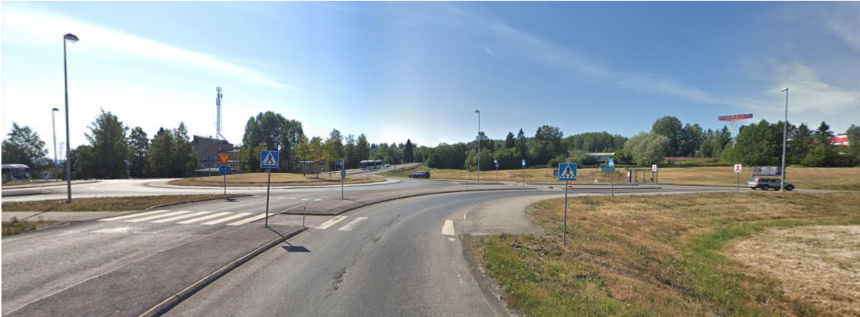
The first roundabout with a separated lane in the view from an arriving vehicle (correlate to figure 4.9).
