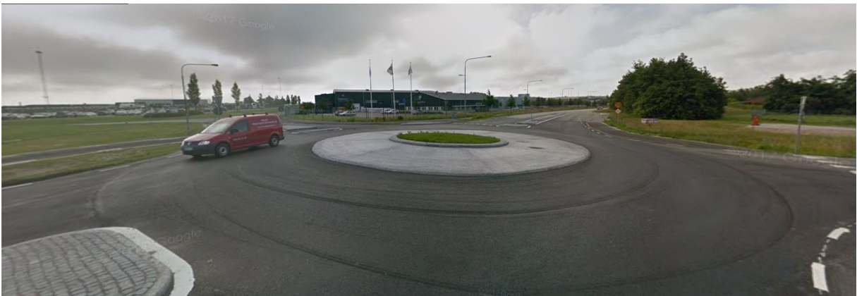
The first roundabout (not visible in figure 4.5 as it has recently been constructed) from the departing view from Malmö (correlate to figure 4.5).
