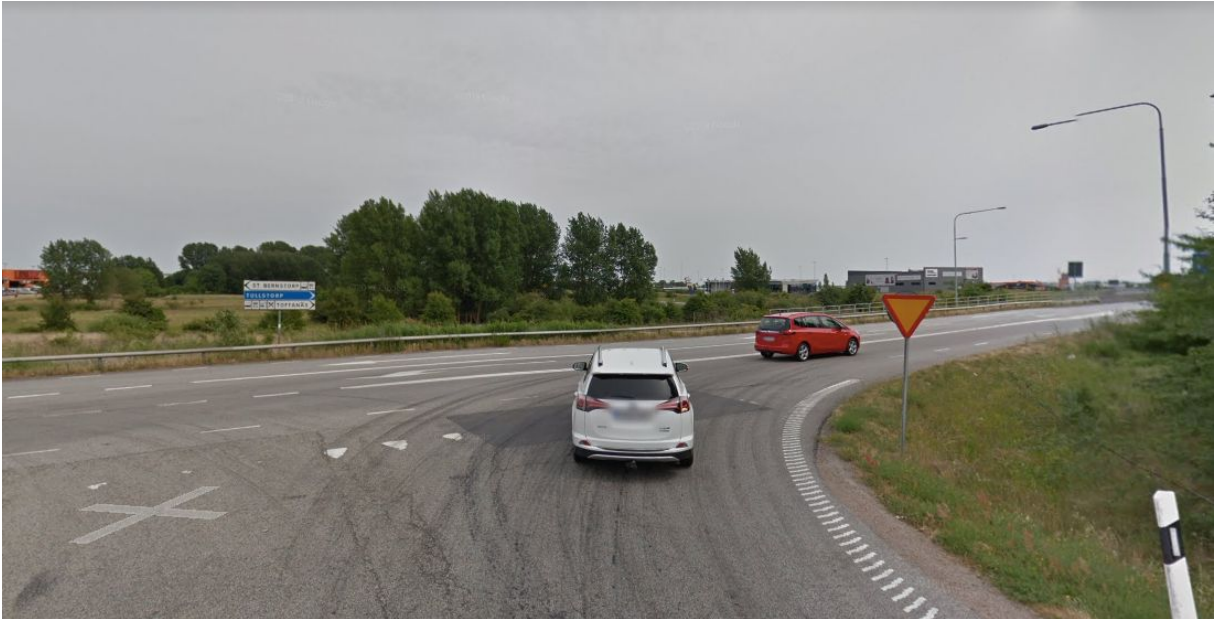
The right turn (exit ramp) to reach the terminal of Malmö from the view of an arriving vehicle (correlate to figure 4.5).
