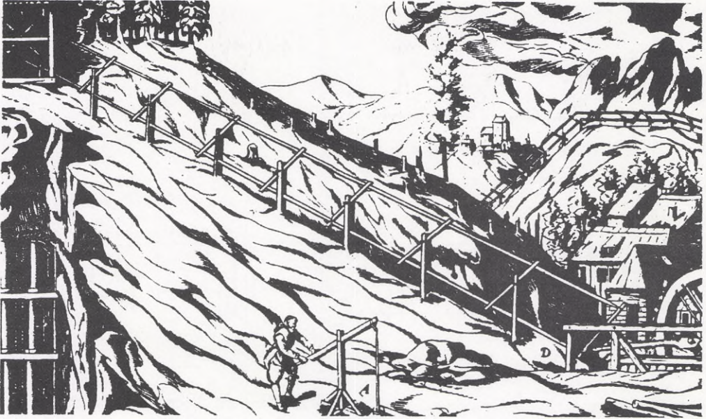
10. Georg von Löhneys 1617: transmission and contouring by means of double rods.
