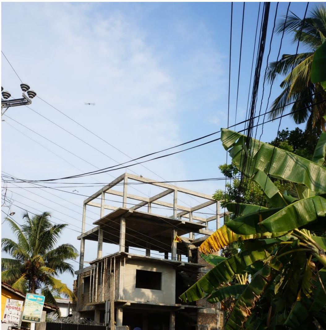
Photo 5. An unfinished hotel construction in Mirissa village. Source: Authors’ own photo.
