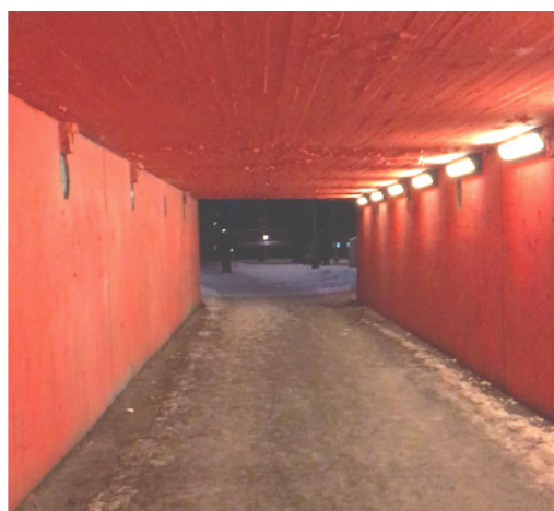
Pedestrian Tunnel of Röda Sten
