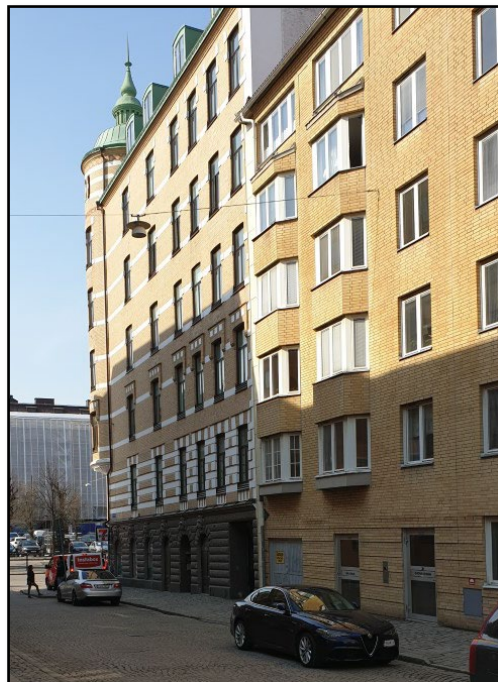
Figure 4.4. The building on the end of the streets shows clear evidence of leaning. Linnégatan 26 in Olivedal. Code: HA1608
