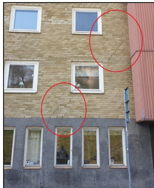
Figure 4.3. A closer look on the damages in the form of sliding bricks on the building at Kommandantsängen. Lilla Risåsgatan 22, Code: KA0110
