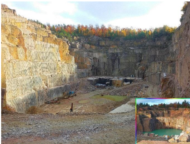
Figure 1 Two photos of open pit mines in Sweden during two stages. The larger photo shows a newly closed mine where water is seeping through the ground and cracks in the wall (darker areas in the middle of the photo). The smaller photo shows a fully developed pit lake
