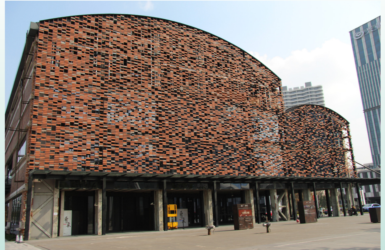
Facade, »Exterior Curtain«, Shipyard 1862 in Shanghai, Kengo Kuma and Associates. Photo: Kristina Fridh.
