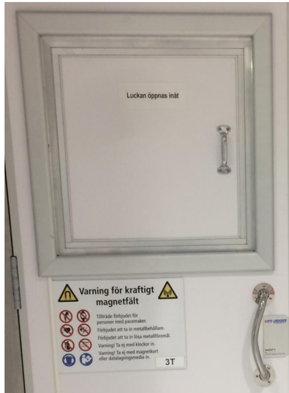
Figure 16. Hatch showing sign stating that it opens inwards.
