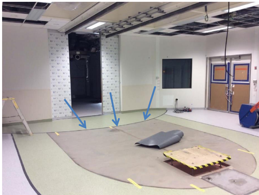
Figure 6. The iMRI Hybrid OR under construction.
