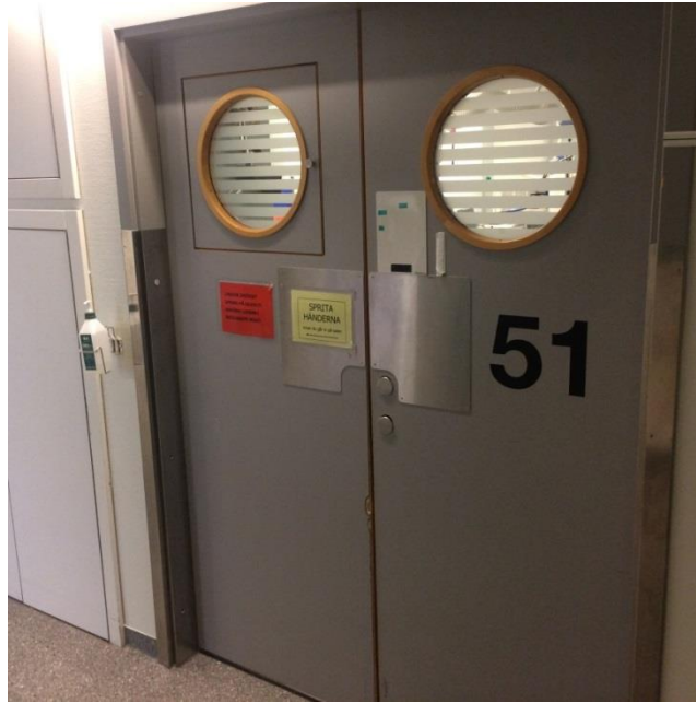
Figure 5. Hatch in the operating room door.
