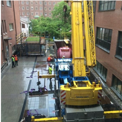
Figure 2. The crane just about to lift the magnet.
