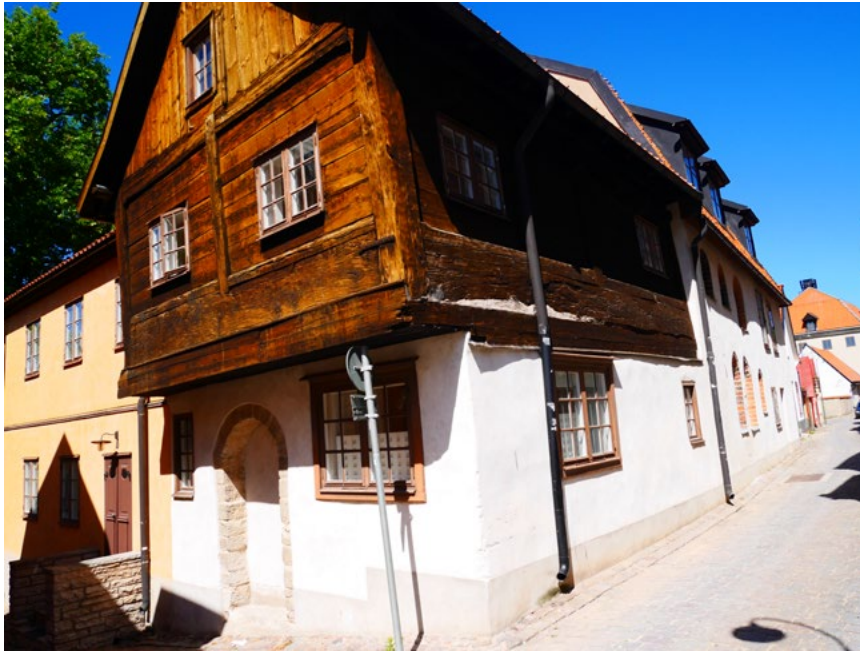
Figure 15 Post and plank building at Mellangatan 35, Visby, Gotland, Sweden. Photo A. Nilsen.
