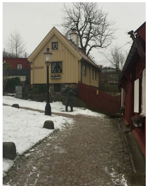
Figure 4 A small building with an over-sized foundation i.e. in this case a substantial cellar. In Gatenhielmska reservatet, Gothenburg. Photo: A. Nilsen
