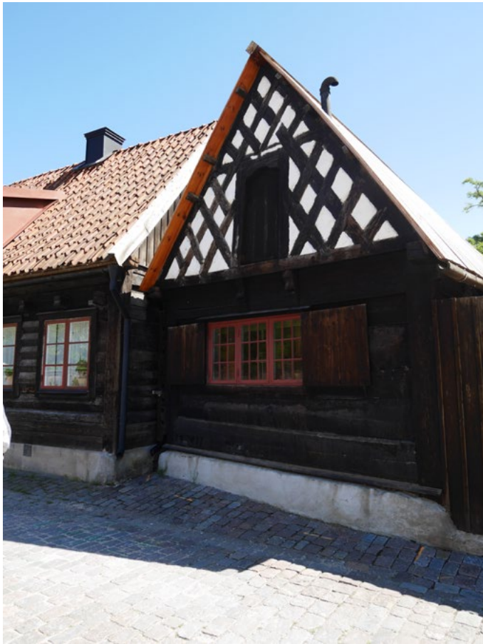
Figure 17 Post and plank building in Mellangatan 4, Visby, Gotland, Sweden. Photo A. Nilsen.
