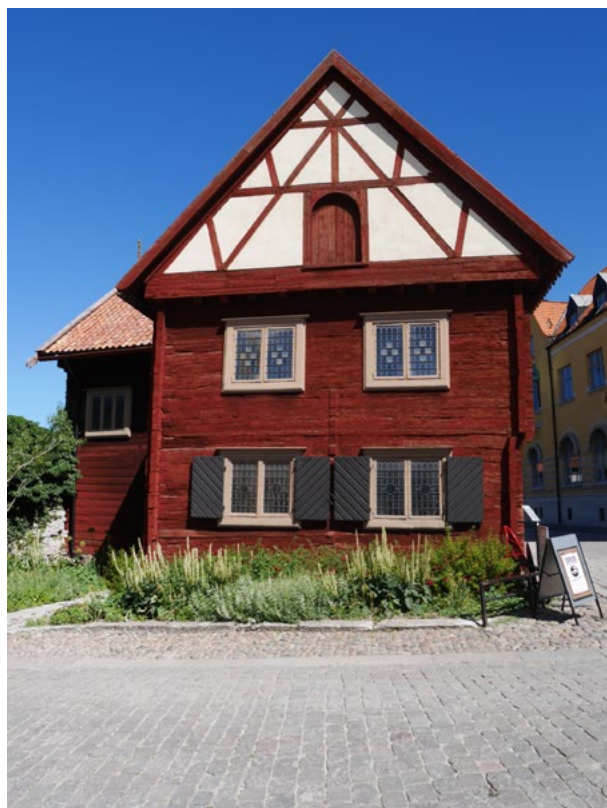
Figure 30 The Burmeisterska log timber house with a timber-framed gable in Visby, Gotland. Photo A. Nilsen
