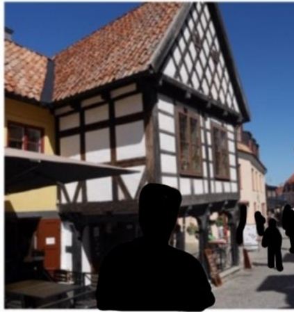
Figure 31 Laboratorn 4 photographed from the front with the verge and of the sidewall with the jetty connected to the property on the other side of the street, in Visby, Gotland. Photos A. Nilsen
