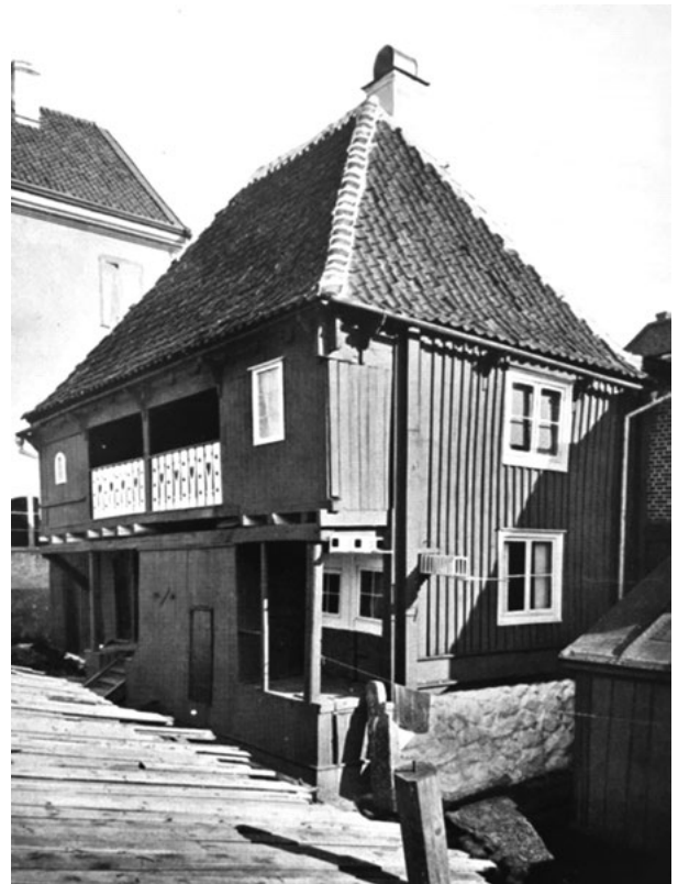
Figure 7 Vinbergska gården, Karlshamn. A house with a balcony that is supported by posts (Bäckström and Wallin 1911, 15).
