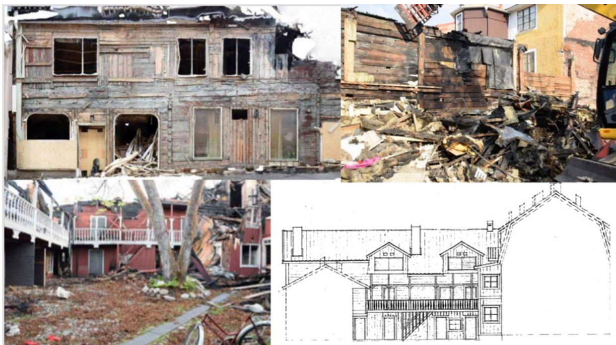
Figure 29 The image at the top left shows the patchwork construction behind the panelling. The image at the top right shows the post and plank construction. The two images in bottom depict the inner courtyard with balconies in Forsselliska gården in Eksjö. (Börjesgård 2017).
