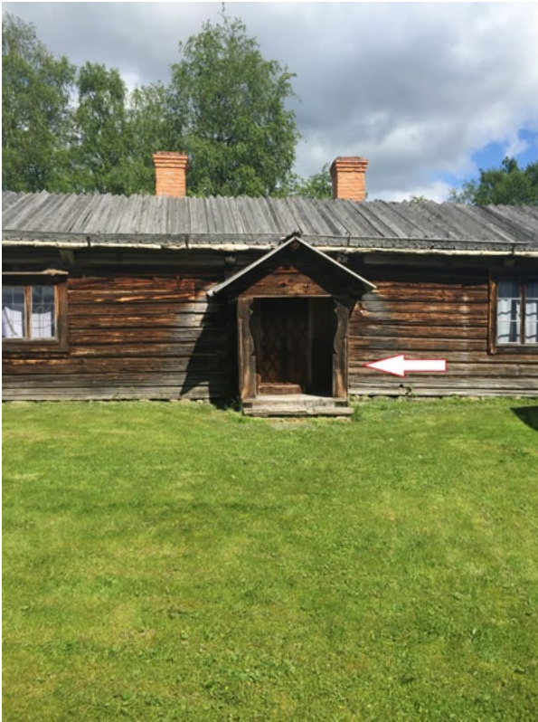
Figure 6 Bislag or porch i.e. a covered superstructure often including a bench to sit on, either side of the entrance.
