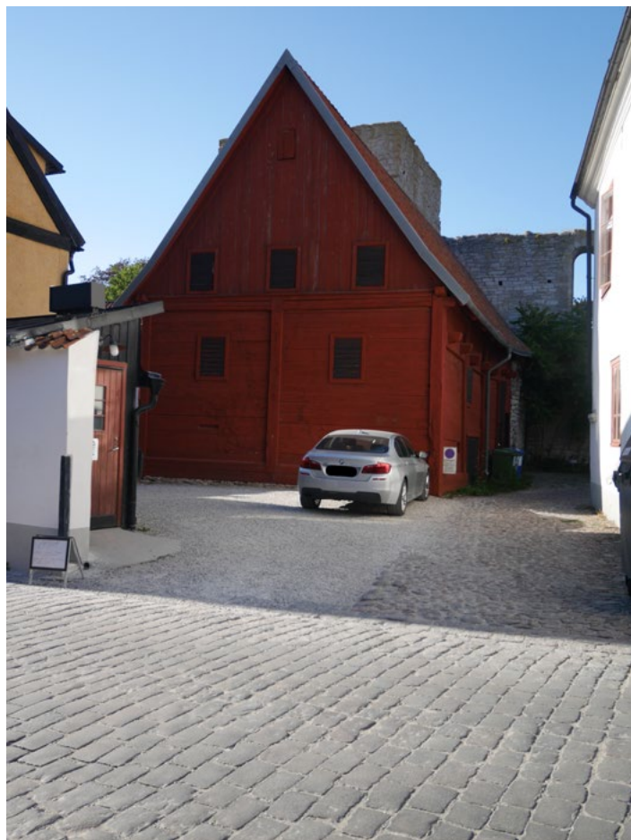
Figure 20 Post and plank building in Visby, Gotland, Sweden. Photo A. Nilsen.
