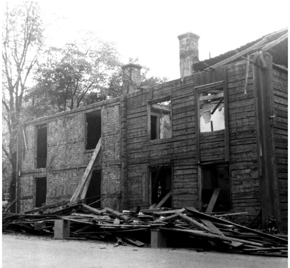
Figure 18 Tideholmsgården in Karlstad was partly built in timber-framing. Photo Gösta von Schoultz, Värmlands museum.
