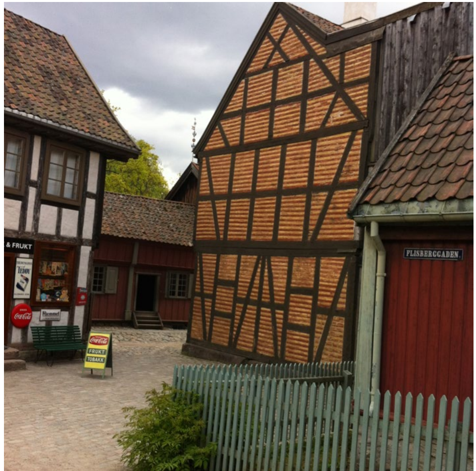
Figure 43 A timber-framed house from Christiania in Norsk Folkemuseum (The Norwegian Museum of Cultural History) in Oslo. Photo: A. Nilsen
