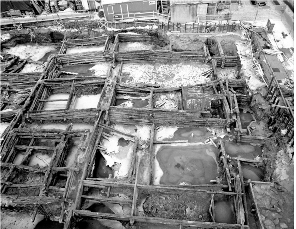
Figure 1 A system of box revetments emerged during excavations in Kv. Ansvaret 1984-1985, Jönköping
