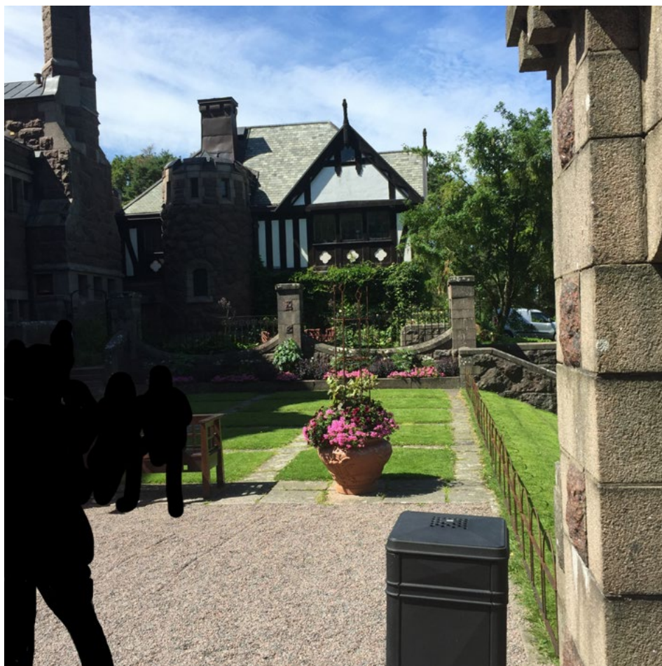
Figure 44 Images of the gatehouse at Tjolöholm in Sweden with an example of close studding. Photo: A. Nilsen.
