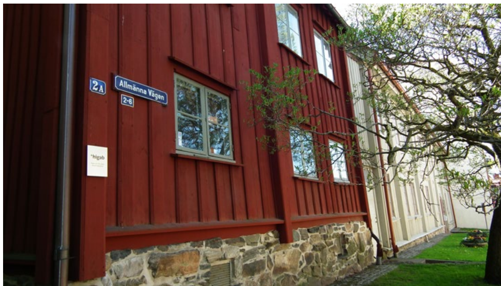
Figure 14 Dahlströmska huset (red). See how it connects to Jedeurska huset nextdoor (with a white facade) Photo A. Nilsen
