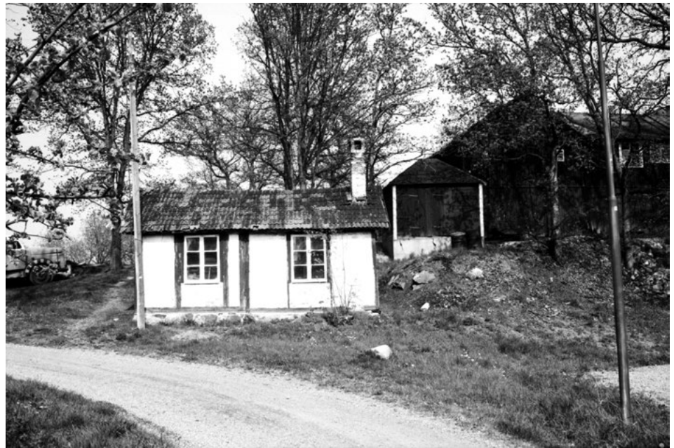
Figure 24 A small timber-framed building in Vrena, Nyköping. Photo Ulla Walukiewicz. Sörmlands museum.
