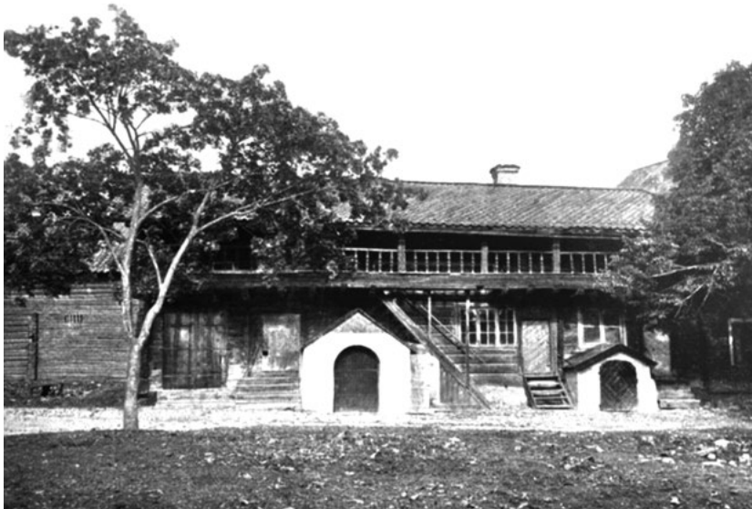
Figure 9 Kungsstugan, Örebro is a two-storey building with an open gallery and a staircase (Curman et al. 1908, Häfte 1, 1908:33).
