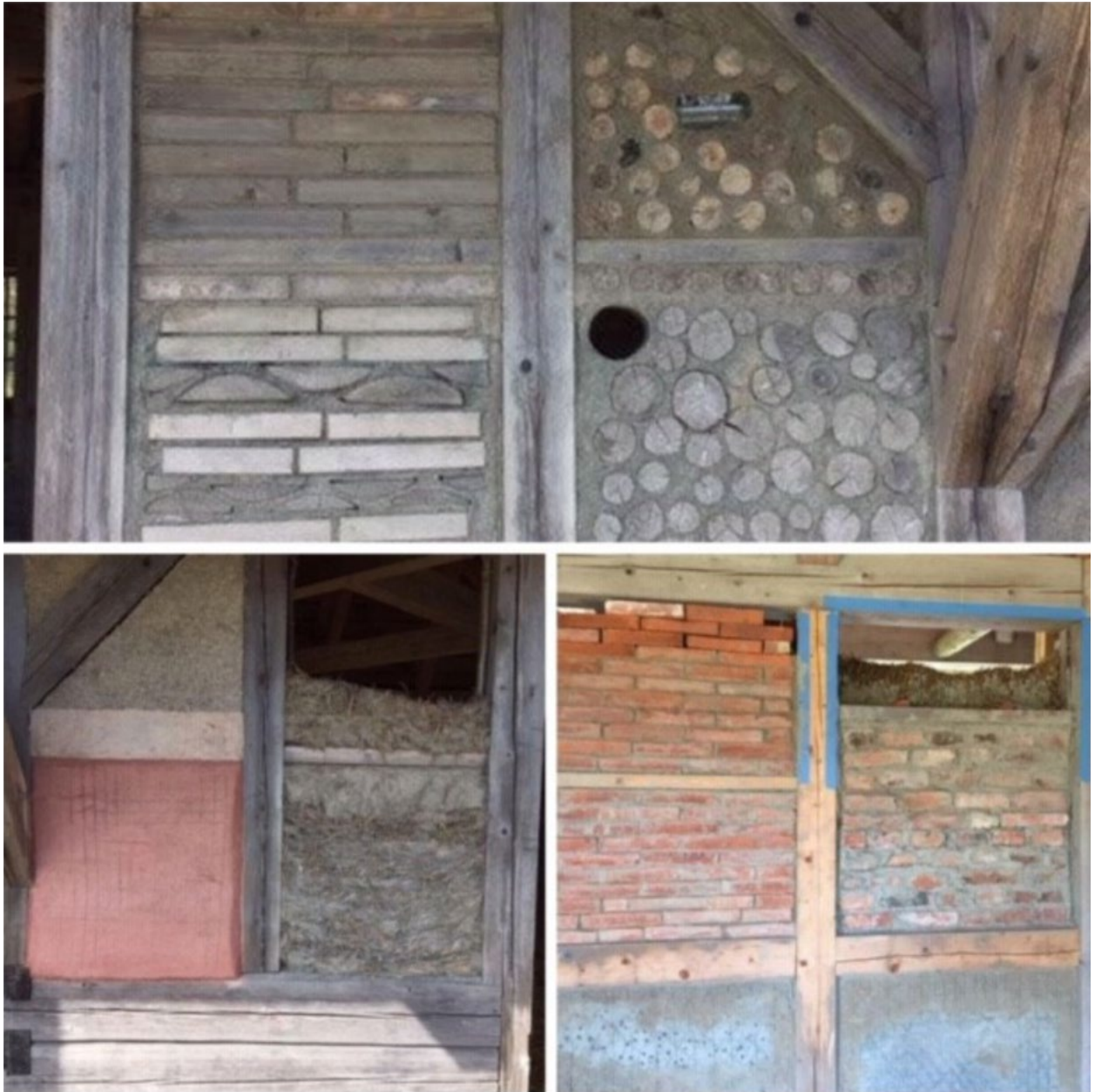
Figure 42 The infill used in timber-framing can come from an array of sources i.e. brick, wattle and daub, logs, rubble and mortar or limestone. Slöjd and byggnadsvård, Nääs Slott. Västarvet, Västergötland. Photo A. Nilsen.
