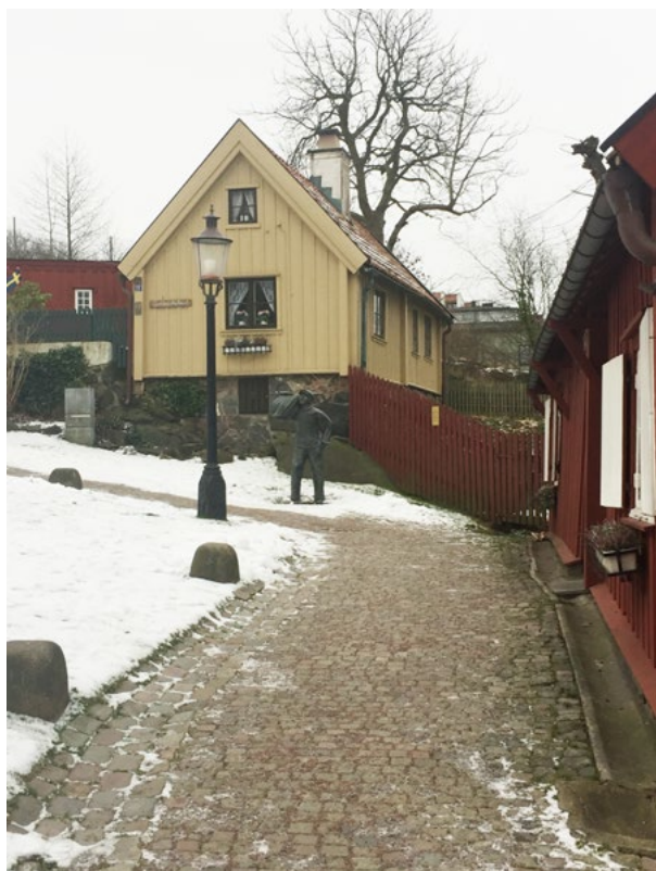
Figure 2 As an example, see this small wooden building on top of a substantial cellar. Gatenhielmska reservatet Gothenburg. Photo: A. Nilsen.
