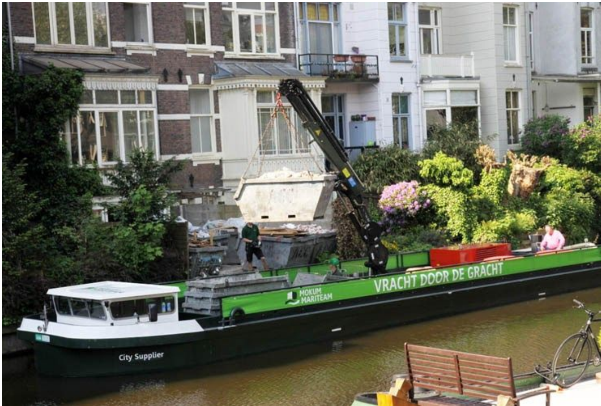
Figure 5: Mokum Mariteam full-electric barge with own crane loading construction waste (amsterdamsebinnenstad.nl)
