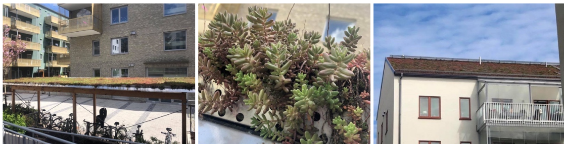
Figure 1: Shows sedum-covered bicycle racks on the far left, a variant of sedum vegetation in the middle and an image of a residential house with sedum roof on the far right. Photo by: Amanda Bäck.
